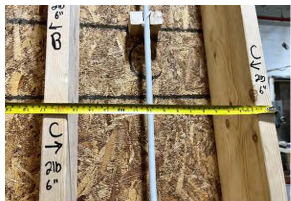
PEX hose at cavity midpoint
