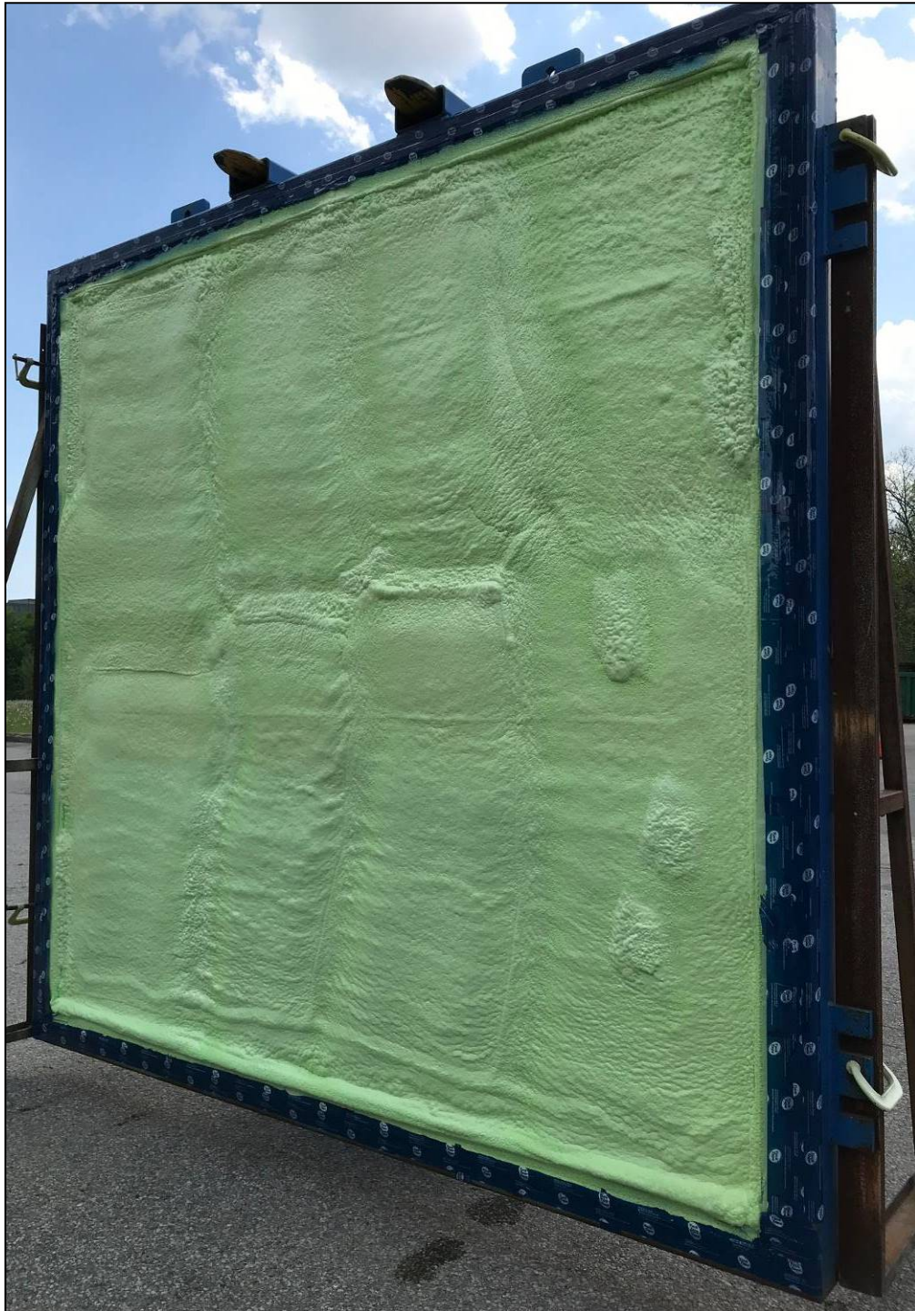
Photo G2 – Air barrier applied onto sheathed wall
