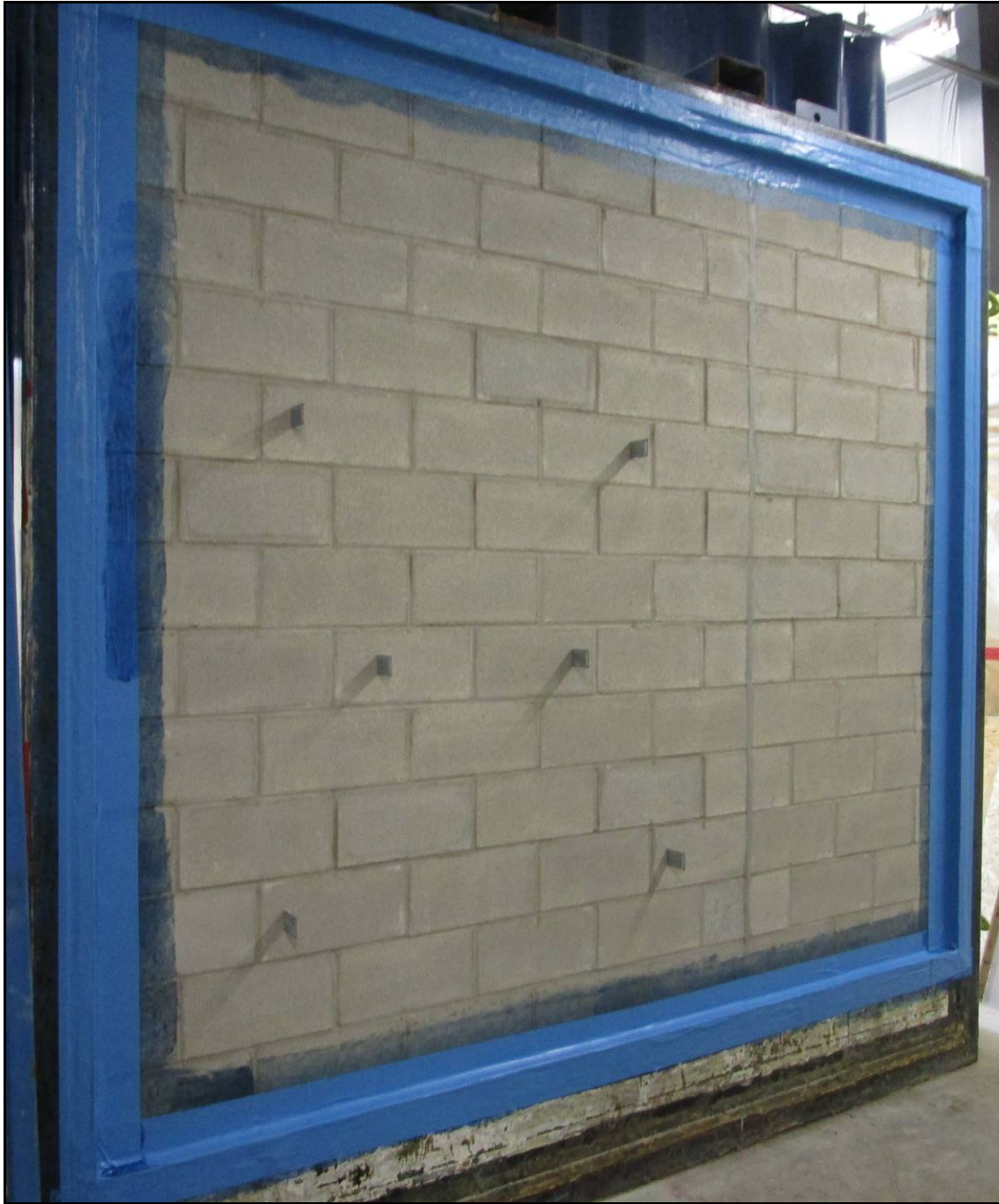
Photo L1 – Penetrations wall section; wall perimeter and foundation interface prepared with membrane and prior to product application
