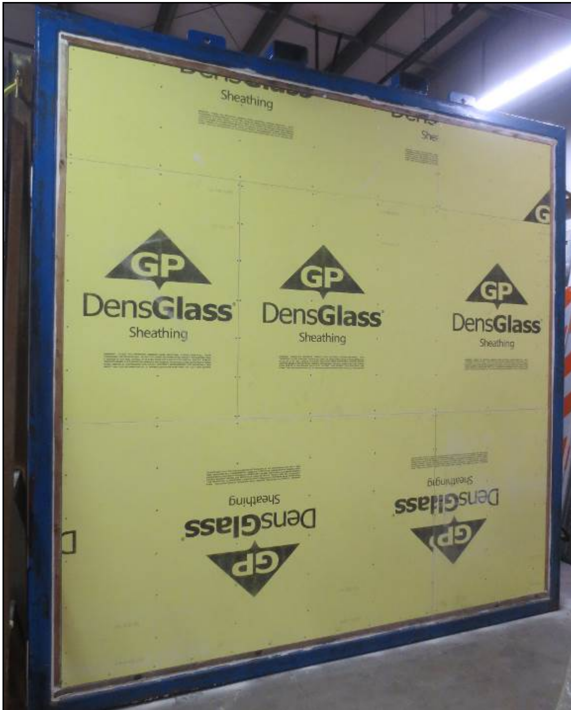
Photo G1 – Opaque steel stud wall section prior to product application
