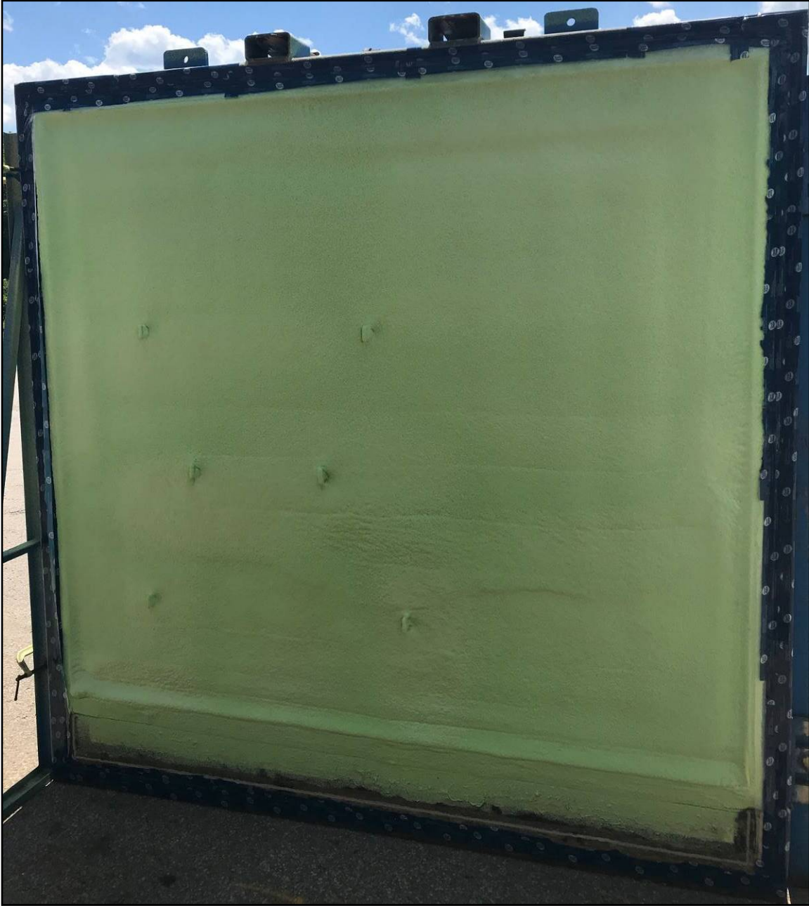
Photo L2 – Air barrier applied onto CMU wall
