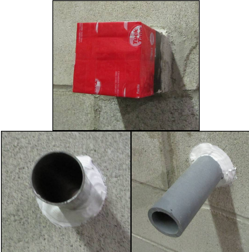
Photo K3 – Penetrations sealed with sealant
