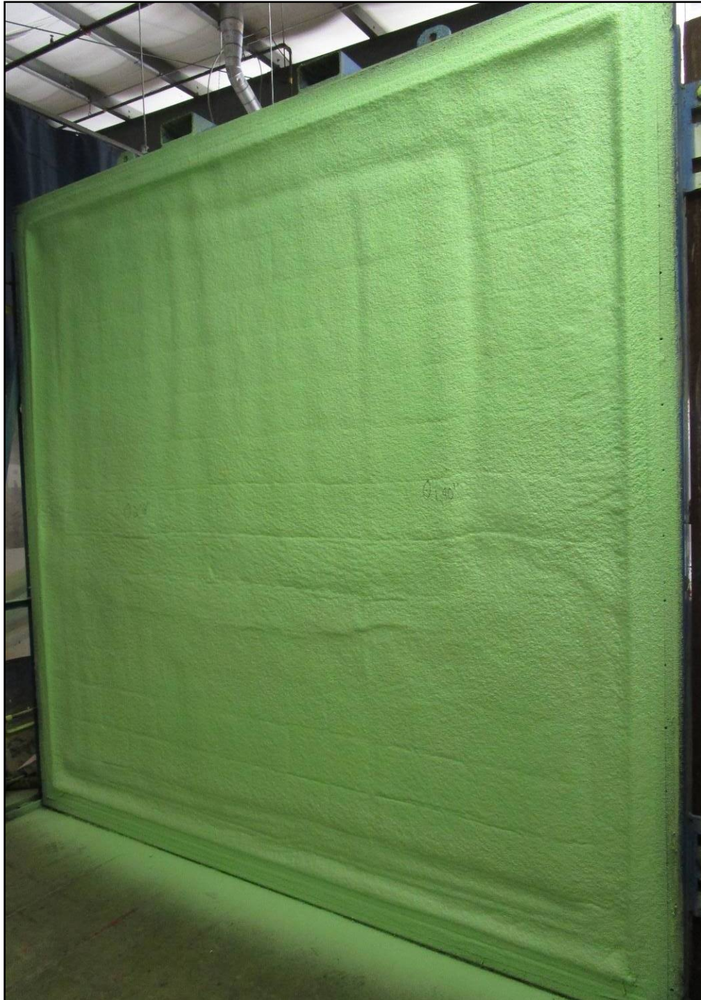
Photo J2 – Air barrier applied onto CMU wall
