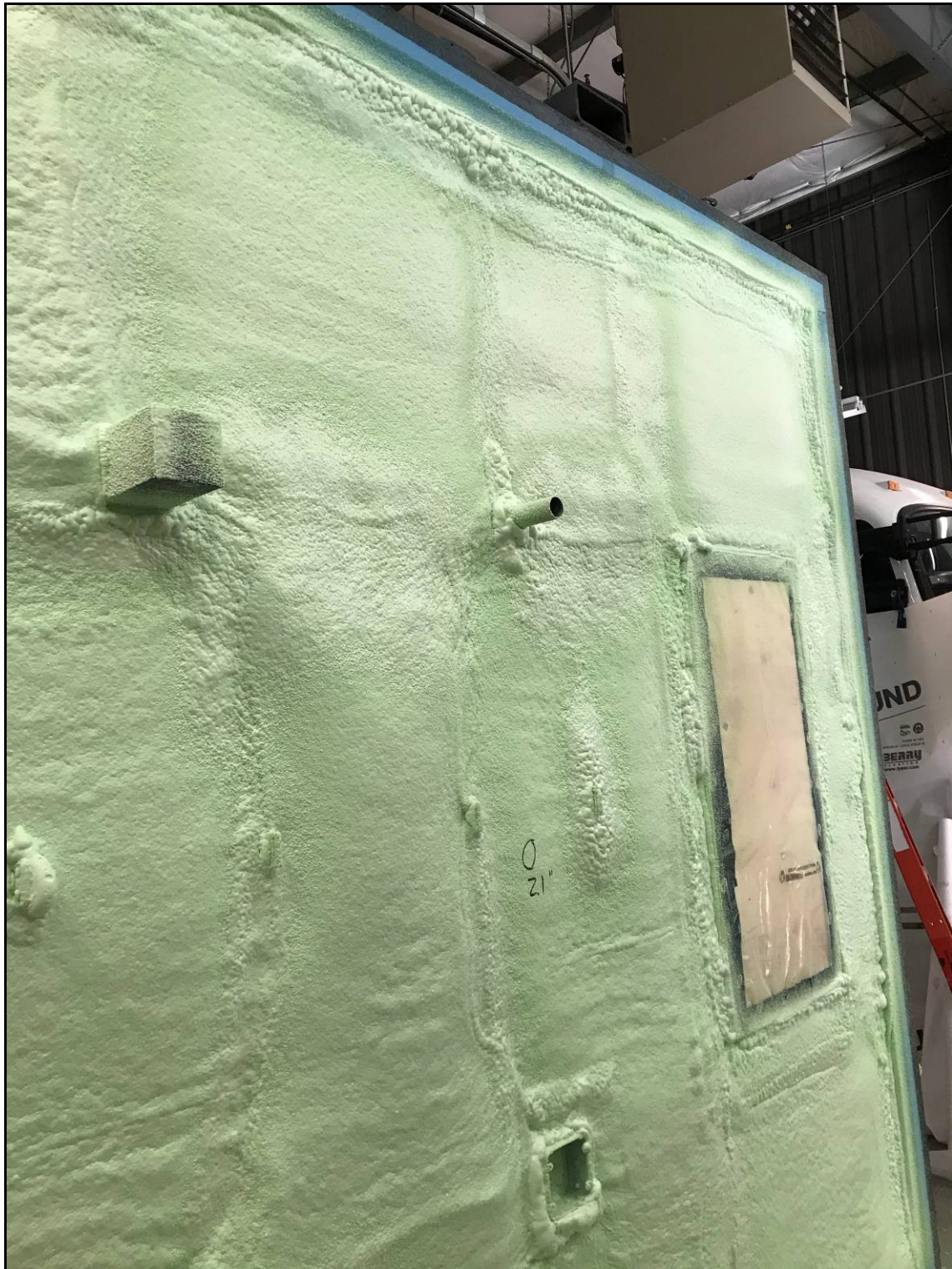
Photo H3 – Air barrier applied onto sheathed wall
